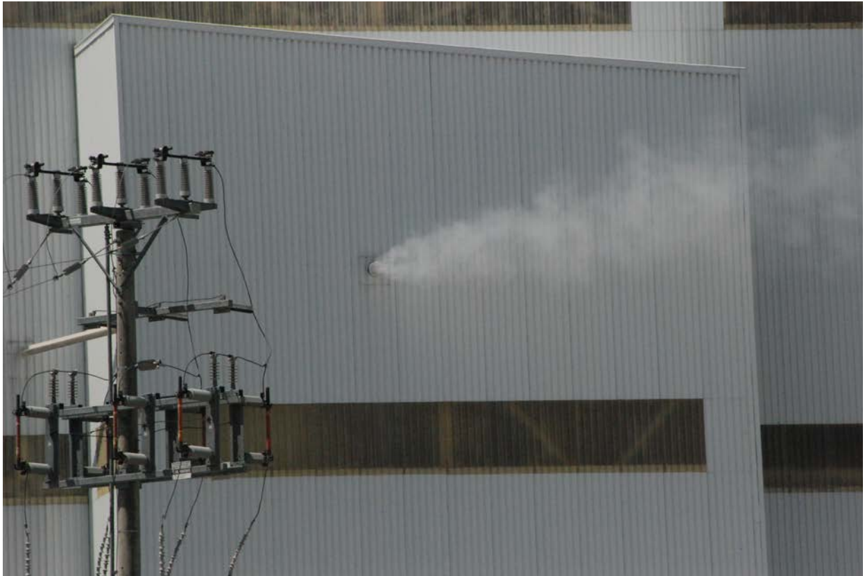
Figure 2 Particulate Discharging from side of plant wall at Blue Mountain Mine
